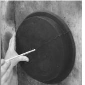
After nailing end cap to form, drive (threaded rod\*) through the end plate and form and (thread nut\*) on other side. **Note**: Remember to measure the (threaded rod\*) to match the length of the sleeve.
