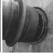
3. Place the Century-Line® Sleeve on the end cap. When field cutting non standard CS sleeve lengths, the sleeve and endcaps total length should be one-fourth (1/4") longer than the thickness of the wall. Note: To insure minimum water migration, center the water stop in wall by cutting equal lengths from each end of the sleeve, except as noted below.
