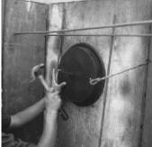
1. Measure the center line to position Century-Line<sup>®</sup> Sleeve end cap.
